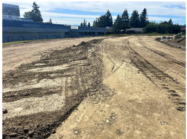
Material from the west end placed and compacted on east end
