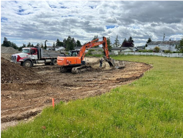
Excavator cutting the west side slope for fill on the east end
